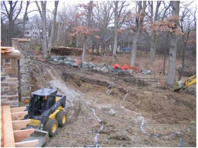
2.) Large scale stone was used to compliment the size and style of the home. The use of properly scaled, individually selected pieces of stone required a large excavator to set. The meticulous facing and placement will allow future plantings to soften and enhance the stonework.
